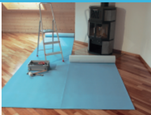
Must be put in place with the edges overlapping.
