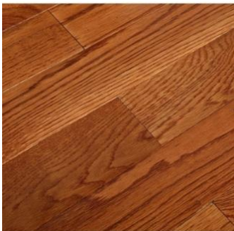
Figure 1: Installed solid hardwood flooring
